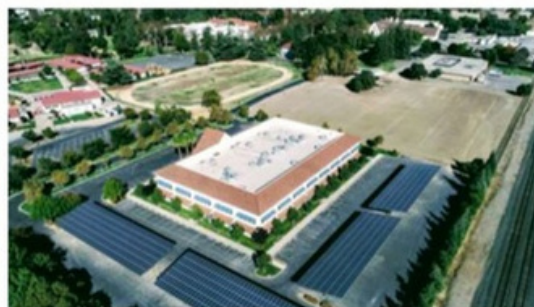
Valley Mountain Regional – 3221kW
