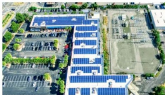
Cost Plus Center – 346kW
