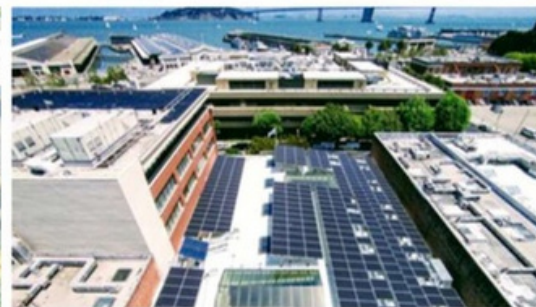
DPR Construction – 118kW
