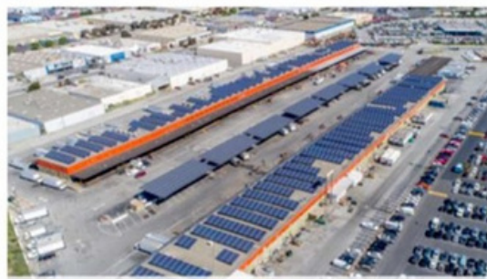
Golden Gate Produce Terminal – 1.32MW
