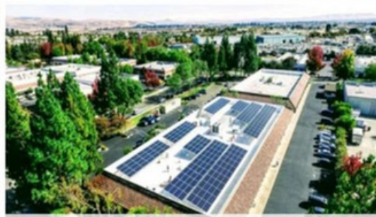
Serpentine Office Park – 100kW
