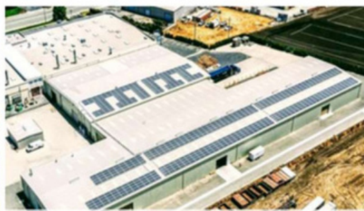
San Benito Shutters – 195kW
